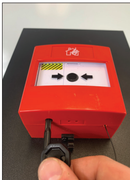
FIGURE 9: RESETTING THE PUSH STYLE CALL POINT
